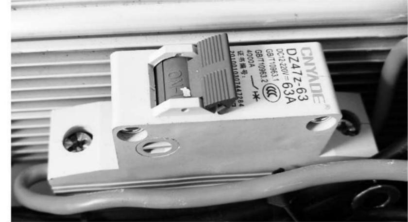
★★ This switch can be protected when there is a short circuit or a severe overload current .
